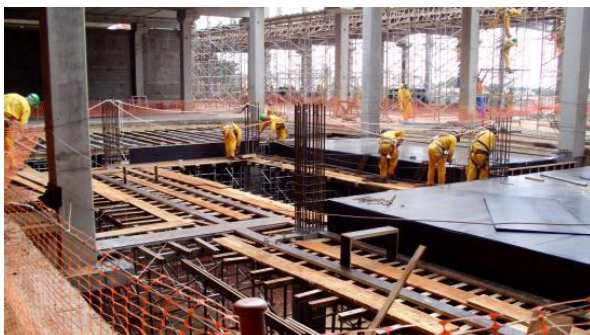
Boulevard Londrina Construction Site
