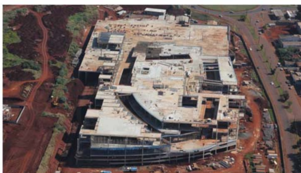
Boulevard Londrina Construction Site
